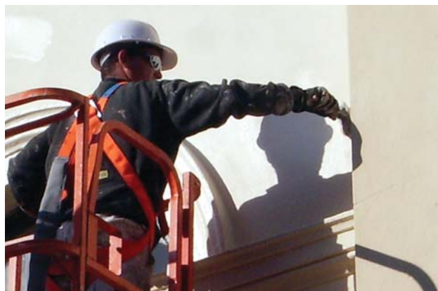
Application of 'the Paint' to the West wall of The Royal Society Building.
